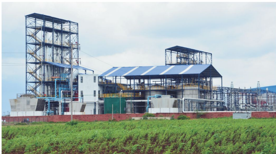
45 KLPD Molasses Based Distillery with Multiple Effects Evaporator for 60% Conc. of Spent Wash
